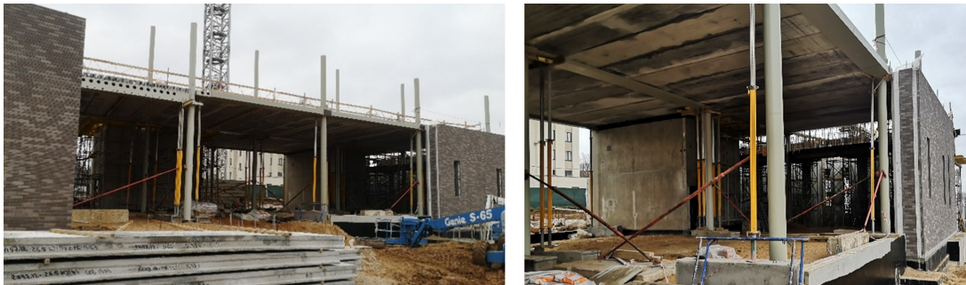
Figure 5. Section 4 – Composite steel-concrete structure
