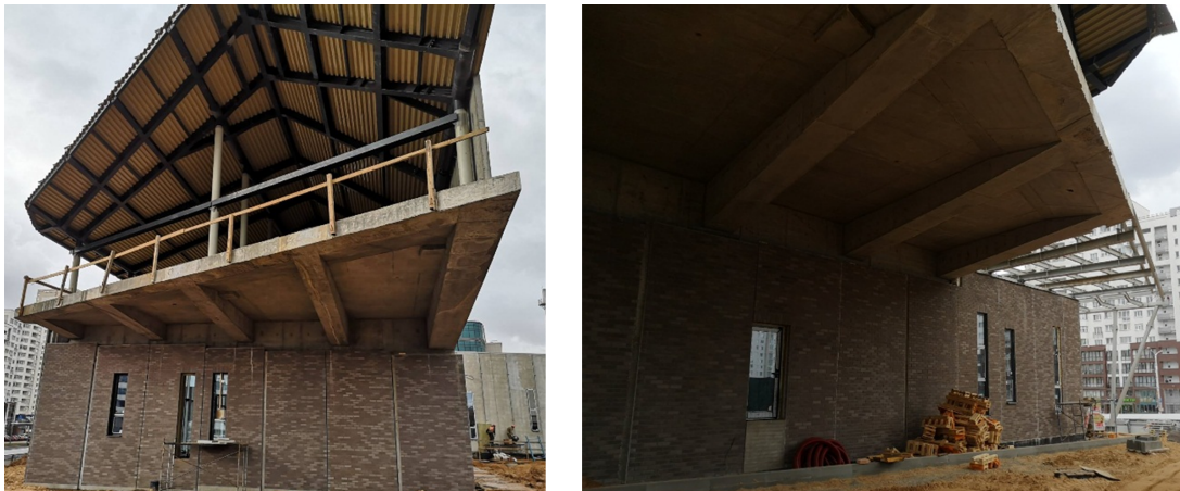
Figure 4. Sections 2, 3 – Post-tensioned monolithic cantilever sections
