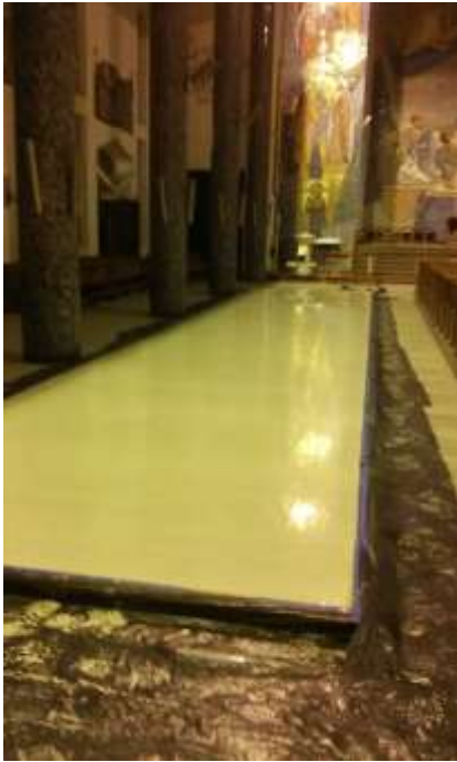
Photo 19: Installation of underfloor heating in the Church of the SHoJ in Gdynia in the rooms of the so-called of the upper church: a), b), c), d), e), f) stages of work (photo by Jacek Bramorski)
