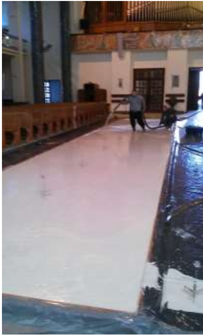
Photo 19: Installation of underfloor heating in the Church of the SHoJ in Gdynia in the rooms of the so-called of the upper church: a), b), c), d), e), f) stages of work (photo by Jacek Bramorski)
