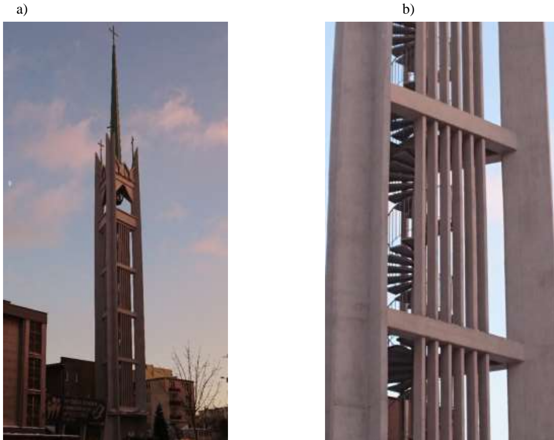
Photo 1. The bell tower of the Church of the SHoJ in Gdynia: a) general view, b) close-up of the internal staircase (photo by Maciej Niedostatkiewicz)
