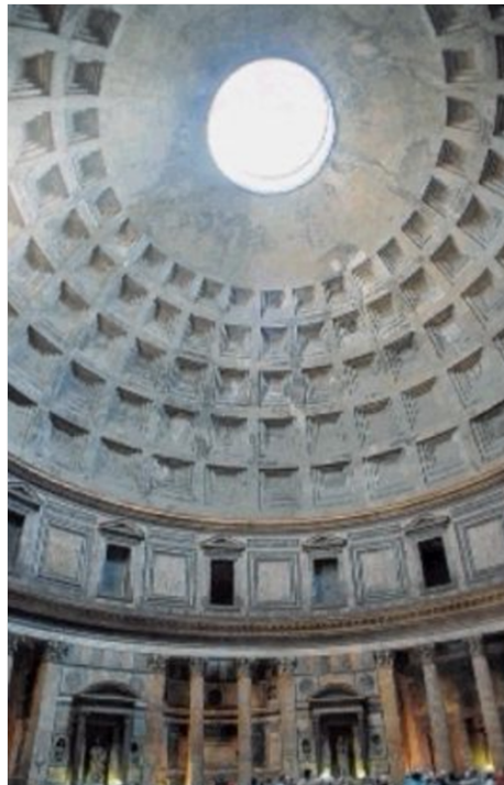
Figure 1. The dome of the Pantheon in Rome with a visible oculus - a central opening with a diameter of approx. 7.9 m [4]
